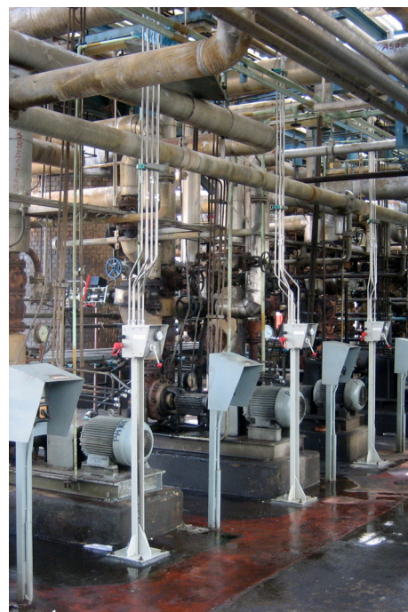
Local operating panel with actuator
